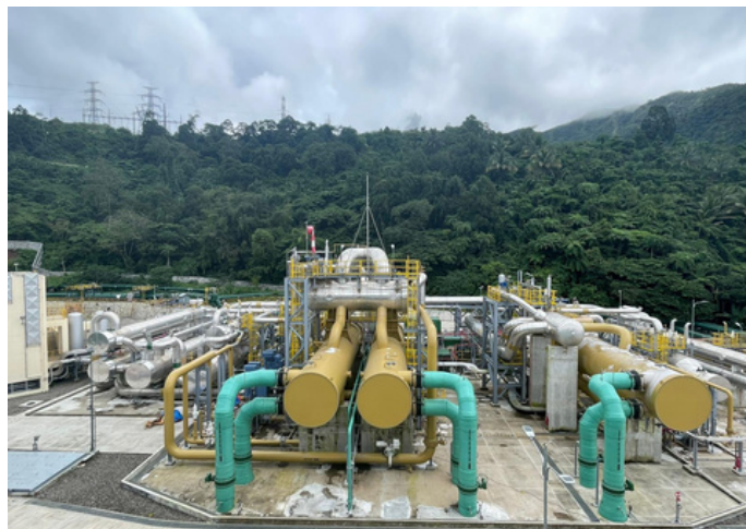
At Mahanagdong in the Philippines, a 24 megawatt binary unit adds generation from lower-temperature brine at an existing geothermal field.
